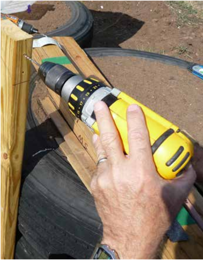
Drill pilot holes prior to attaching bracket. Use 1-inch wood screws to fasten bracket to frame member.
