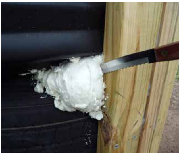
Seal gaps at all four corners of the bed using foam sealant. After the foam cures, use a knife to remove excess.
