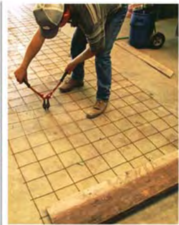
Removing a 48-inch section of mesh from roll
