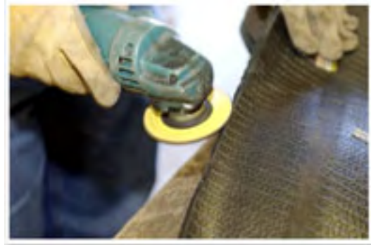
Use a grinder to remove wire stubs
