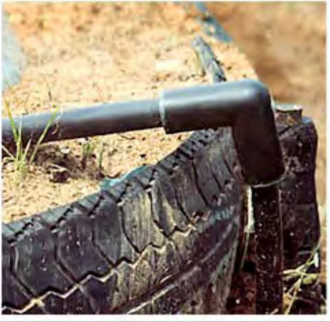
Use an "ell" fitting to connect the main line with emitters.
