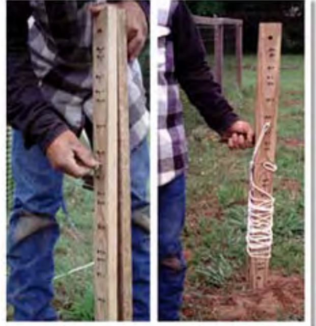
Use a bolt and a wing nut to make the template set transportable.
