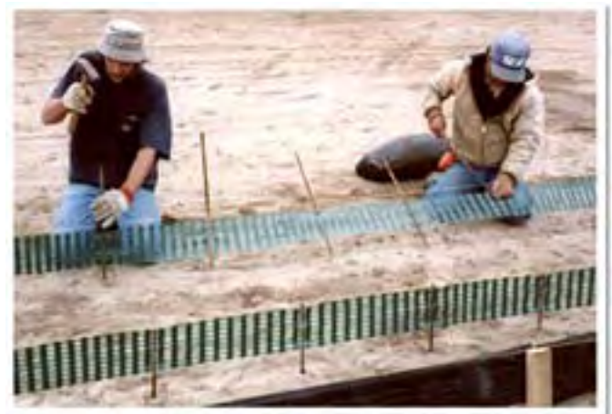
Secure the mesh to the ground with 3/8-inch rebar stakes.
