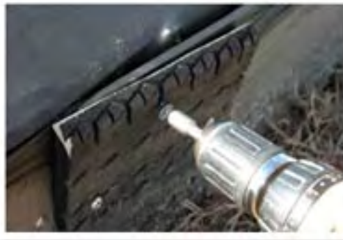
Securing lath to bed wall
