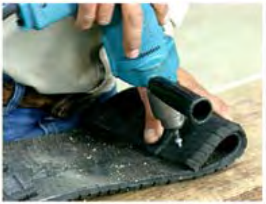
Forming the loop at the end of the board.
