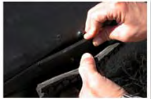
Inserting lath behind pocket
