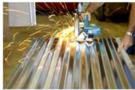
Use of circular saw to cut sheet metal
