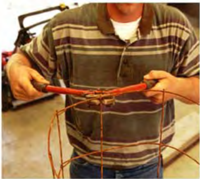
Removing an end rung of wire to form wire "toes"
