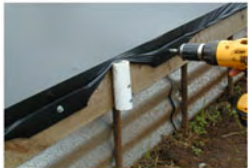
Placement of lath on frame between stakes
