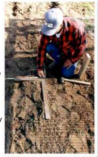
Initial squaring of plot can be accomplished with the aid of a framing square.
