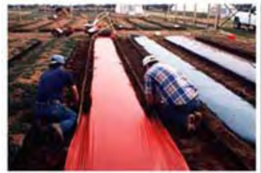
Burying the edges of plastic mulch within the bed using the alternative trench application method.
