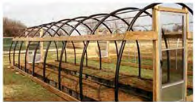
10-foot-wide permanent hoop house built of 2-inch high-pressure polyethylene pipe
