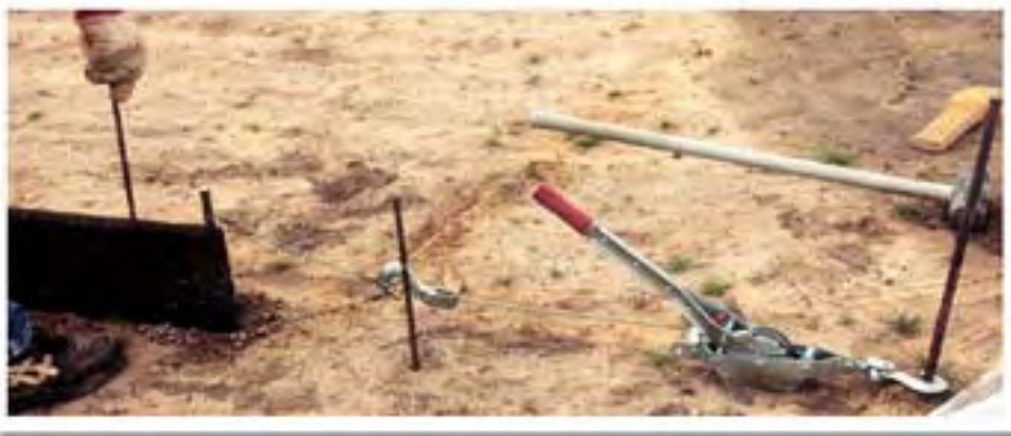
Use a hand winch to stretch 30-foot-long rubber boards prior to staking.
