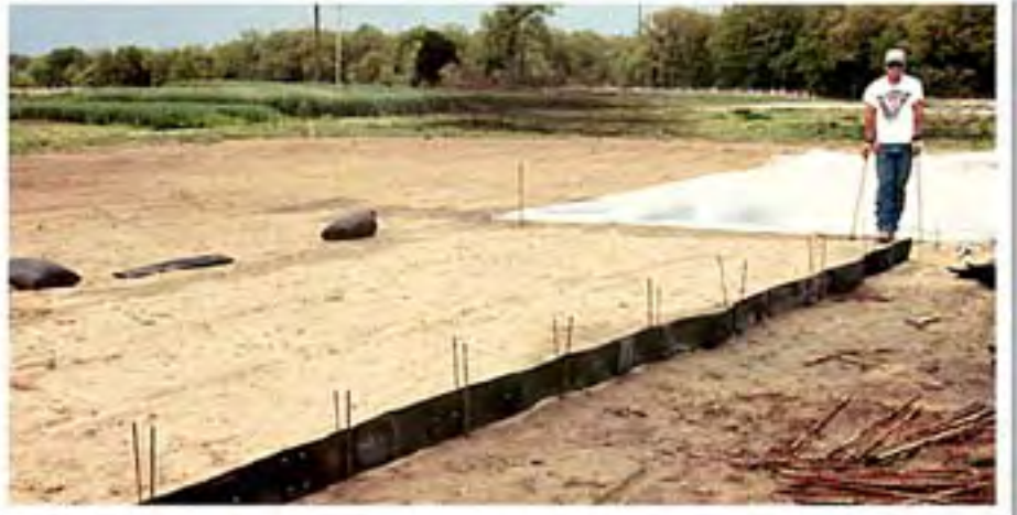
A 30-foot rubber board rests in rebar "cradles".
