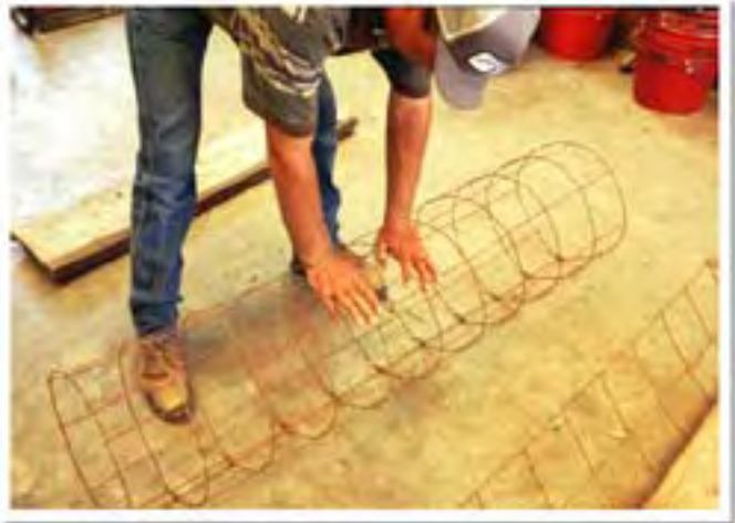
Connecting fingers to opposite edge to form cage
