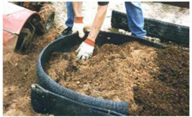
An end piece made from a single piece of tire tread
