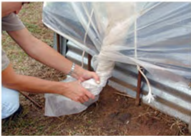
Preparing cover end prior to securing to frame
