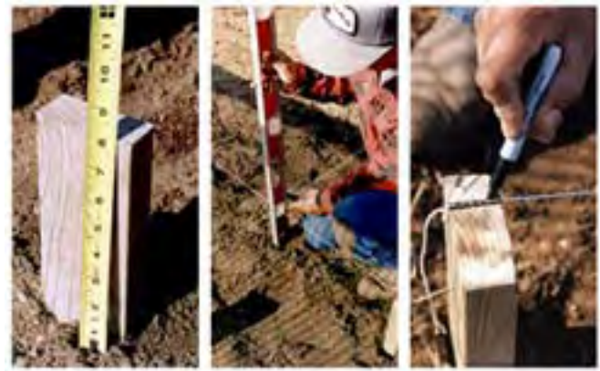
Figure 2. Both A and D stakes should be driven to the same height above ground (not the same elevation), with the height determined by the height of the beds. Because the site is sloped, A and D will be at different elevations. To insure a uniform slope across the plot, use a leveling instrument to level A and B stakes with each other and C and D stakes with each other.
