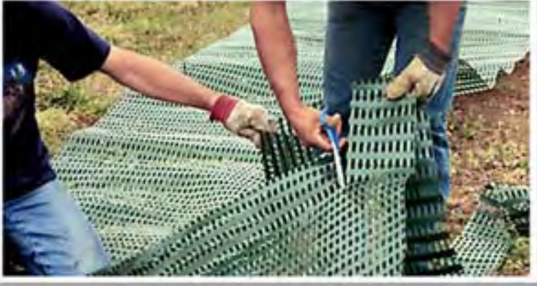
Cutting mesh borders couldn't be easier – household scissors are sufficient to get the job done!
