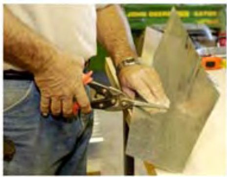
Use tin snips to prepare flashing.
