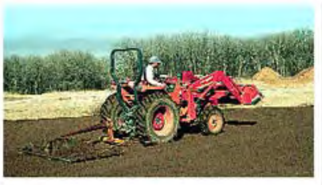
Establish a uniform grade before constructing the garden beds.
