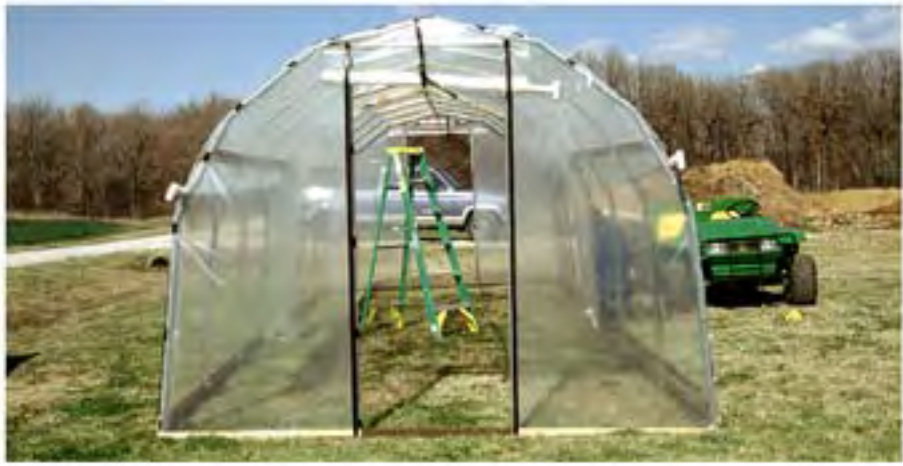
10-foot-wide moveable hoop house equipped with removable end walls and roll-up door
