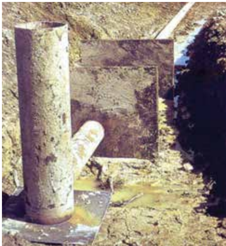
Fig. 3. A drop inlet spillway with anti-seep collars (USDA-NRCS Agriculture Handbook 590 "Ponds – Planning, Design, Construction").
